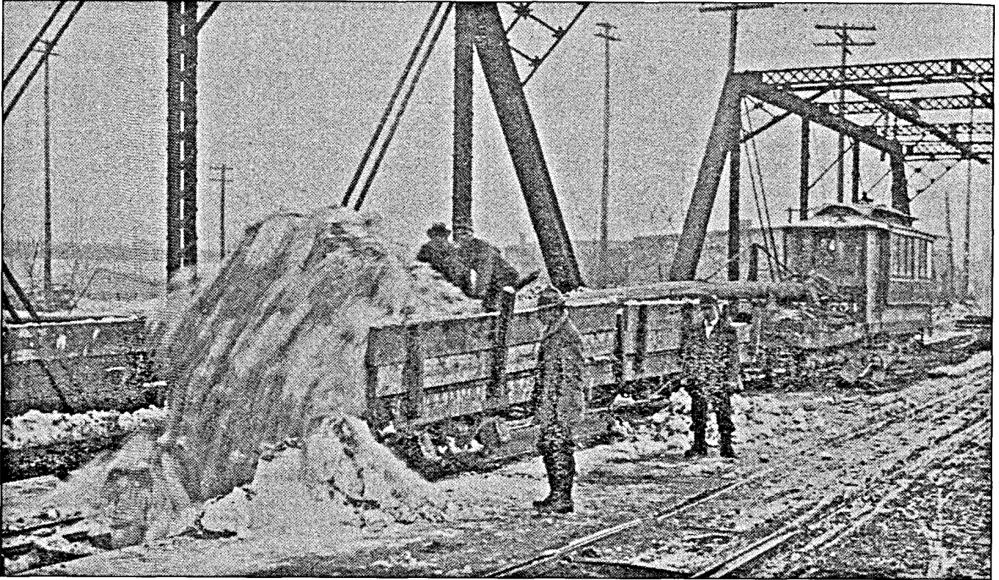
In a piece of creative snow removal, tramway workers loaded snow onto flatcars, hauled the cars to a bridge over the South Platte River, and—with the help of a scraper and long pole attached to a trolley—dumped the snow through a hole in the bridge and into the river.
