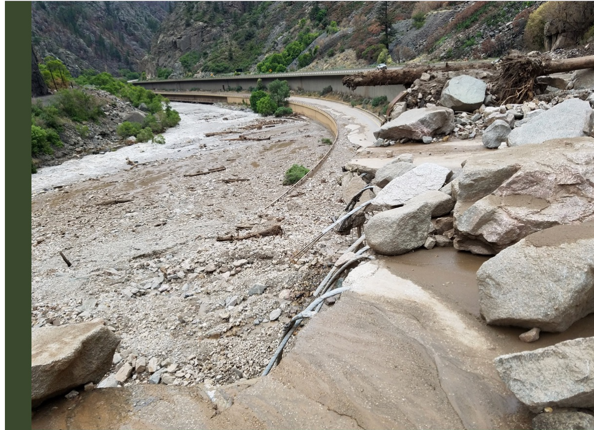
I-70 flash flood and debris flow
