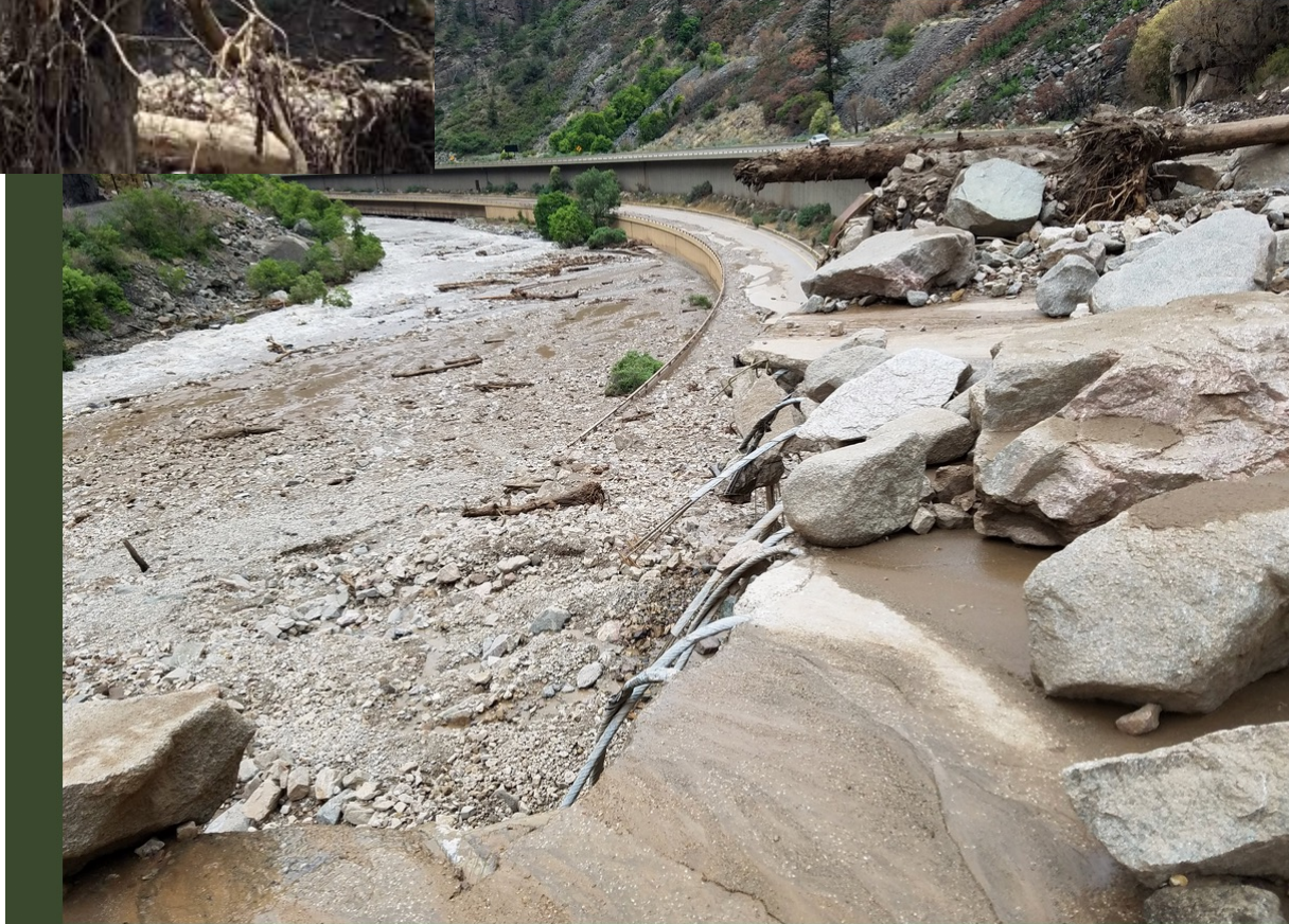
I-70 flash flood and debris flow
