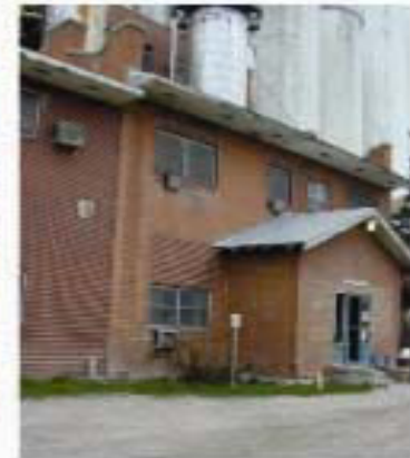
Close up of sensor location
