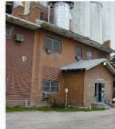
Close up of sensor location
